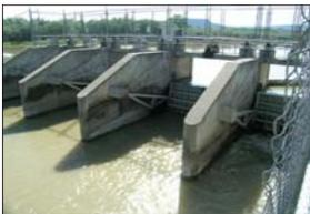
At the diversion dam, the main lateral has a capacity of 90 cubic feet per second (cfs). Project lands are served from turnouts at the major canals and laterals. A number of natural drainage channels that cross the project have been improved to prevent flood damage to project lands and irrigation structures.
