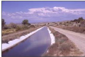
Water for irrigation is diverted from the river above Blanco. The water delivery system consists of a main gravity canal, a hydraulic-turbine-driven pumping plant and an auxiliary pumping plant, three major laterals, minor distribution laterals, and the drainage system.
